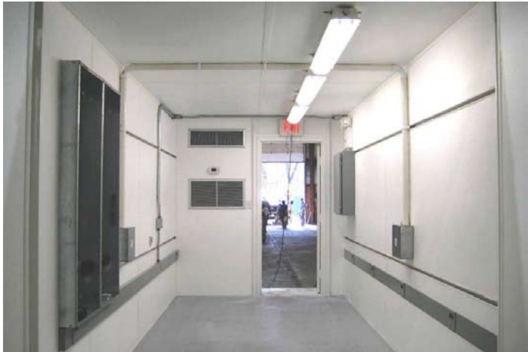
Figure 8. A typical Site Services Building before outfitting with electronics, computers, and other components.
